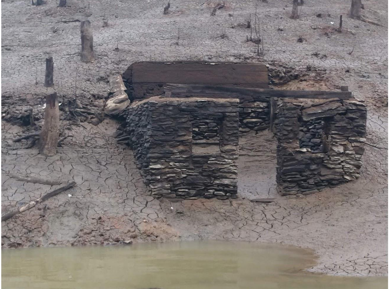
Figure 2 -View of Structure Detail
